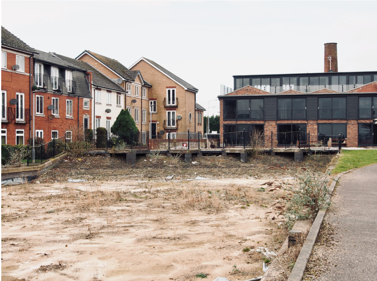
FIG. 5 Silted locally listed slipway, original photo by author, 2020.
