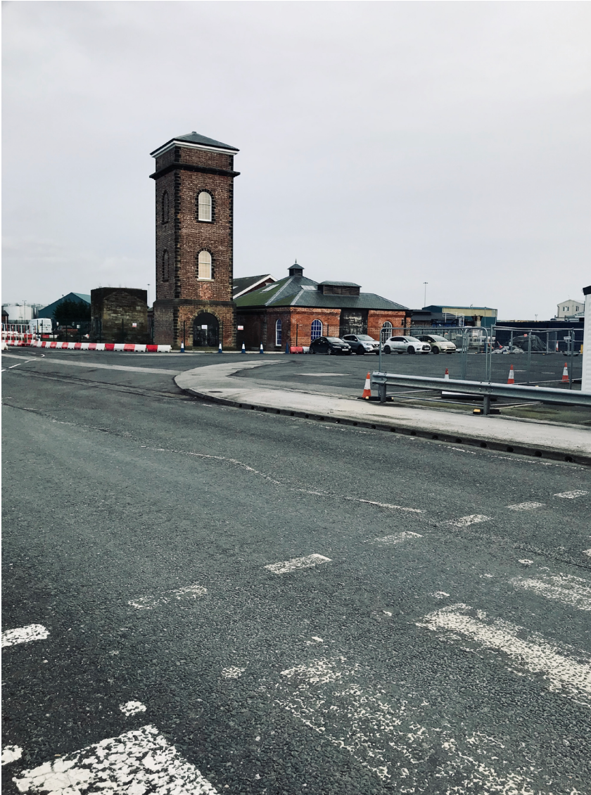
FIG. 8 Grade II Listed Hydraulic Tower and Pump House, original photo by author, 2020.
