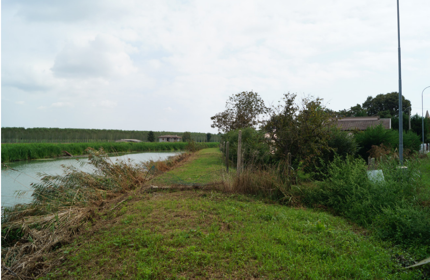
FIG. 11 Messezantica embankment. Credits: Rosa Grasso
