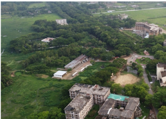
ii. Drone view of campus
