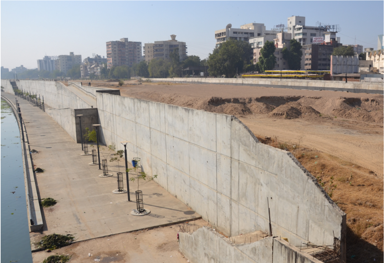
FIG. 6 Land reclamation and construction of RCC retaining walls along the Sabarmati river. View from Gandhi bridge towards the South (photo: Mariana Félix Paisana, 2013).
