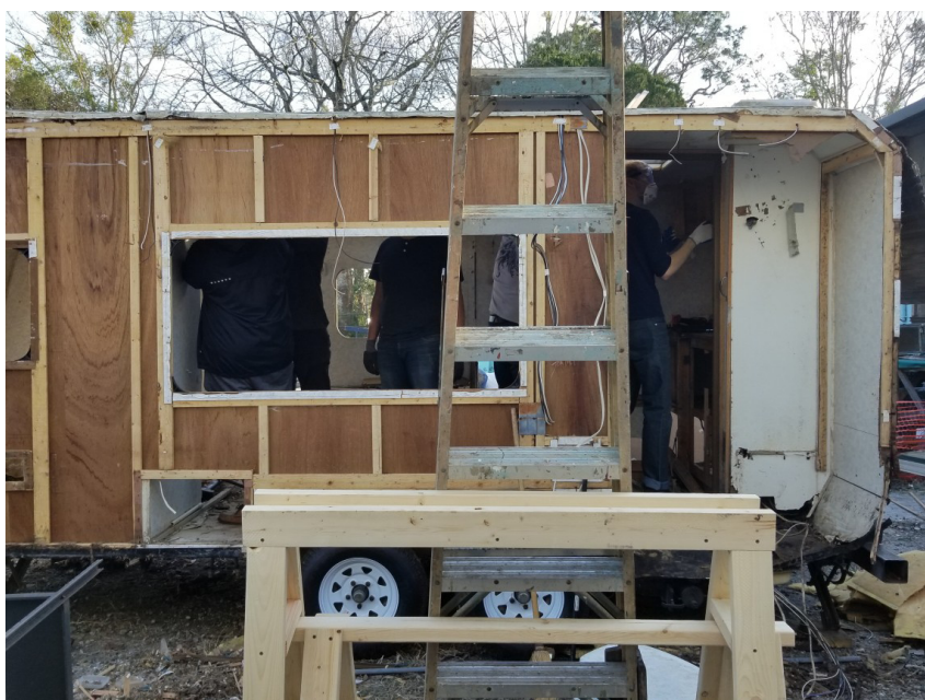
FIG. 6-7 Travel trailer used as the base for the Maker Space, in the process of disassembly
