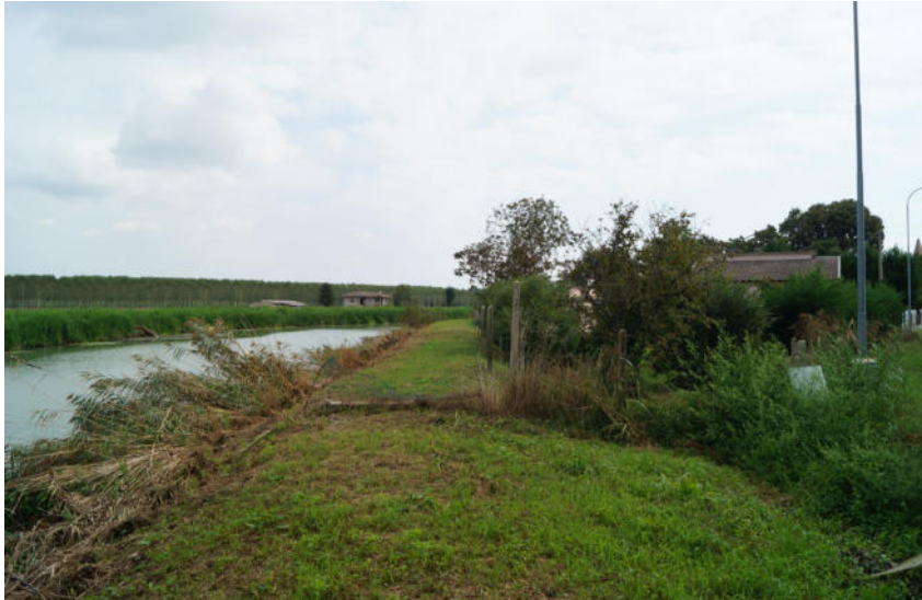
FIG. 11 Messezantica embankment. Credits: Rosa Grasso
