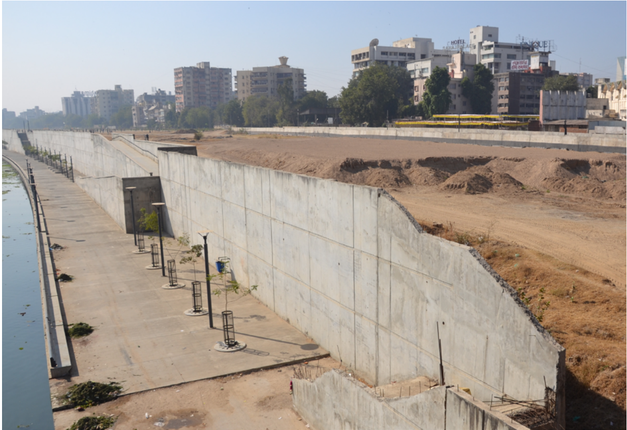
FIG. 6 Land reclamation and construction of RCC retaining walls along the Sabarmati river. View from Gandhi bridge towards the South (photo: Mariana Félix Paisana, 2013).
