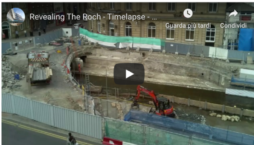
FIG. 2 Time-lapse video of the river Roch deculverting https://youtu.be/x2AQkEG308Y .
