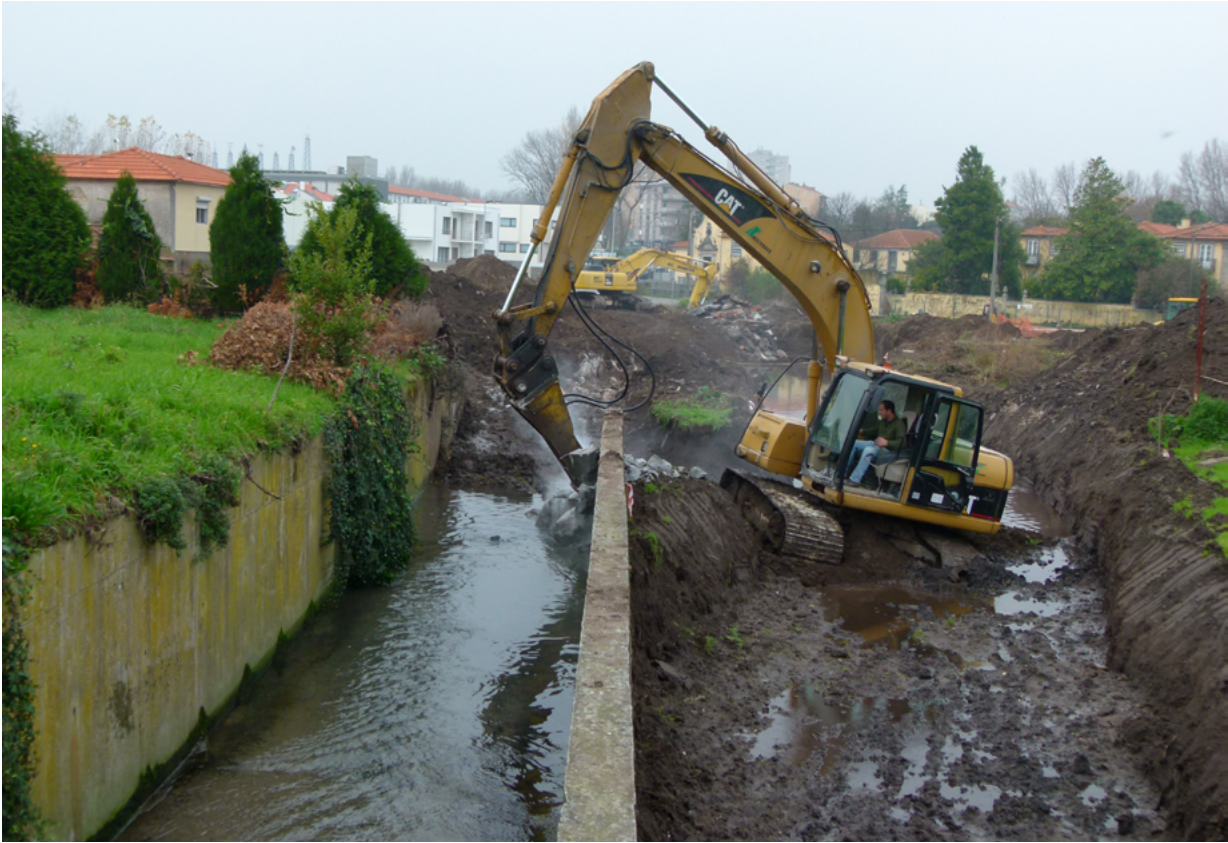
FIG. 1 Dewatering of the Granja stream / source: Águas do Porto (Porto Water Company)
