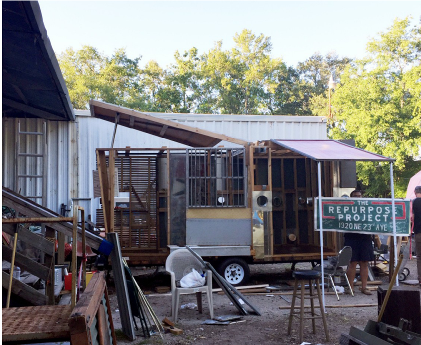
FIG. 9 Maker Space nearing completion, on site at the Repurpose Project
