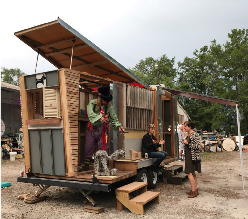
FIG. 10 Maker Space nearing completion, on site at the Repurpose Project
