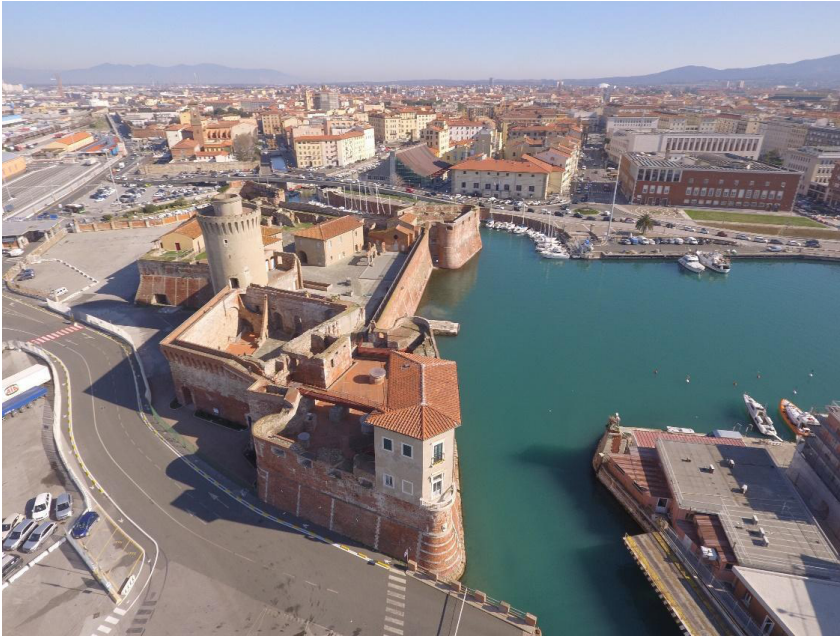
FIG. 5 Livorno's Old Fortress- (Photographic material owned by the North Tyrrhenian Port Network Authority)
